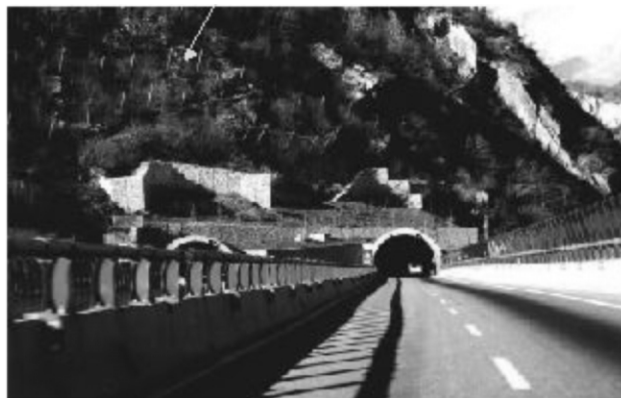
Fig. 7. Ramat tunnel portal with net fences.
