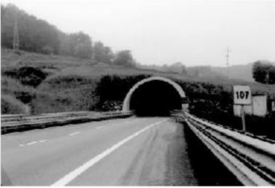
Fig. 4. The arched portal of the Maloni tunnel (Torino side, Turin–Savona motorway).
