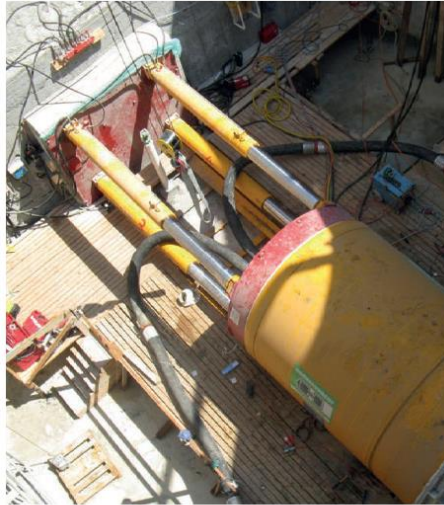
Thrust pit set-up
