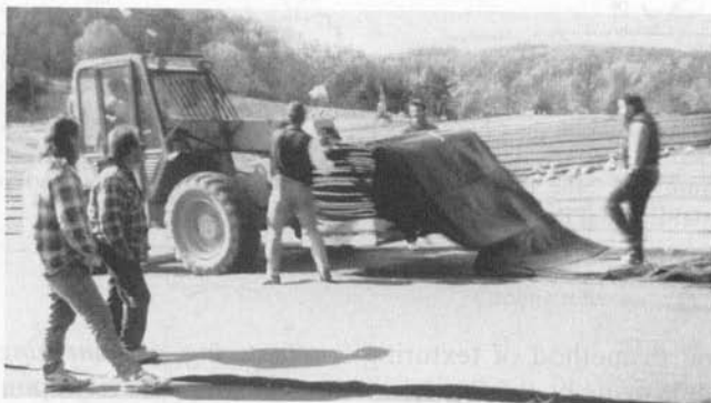
(b) Accordion-folded pallet of calendered polyvinyl chloride
