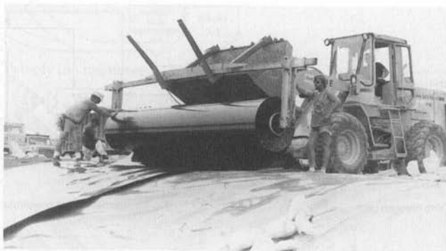
(a) Roll of extruded polyethylene
