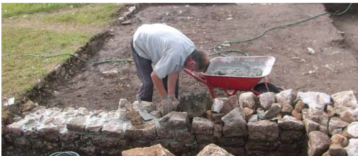
Sl.l Radovi na terenu / Fig. l Works in the field
