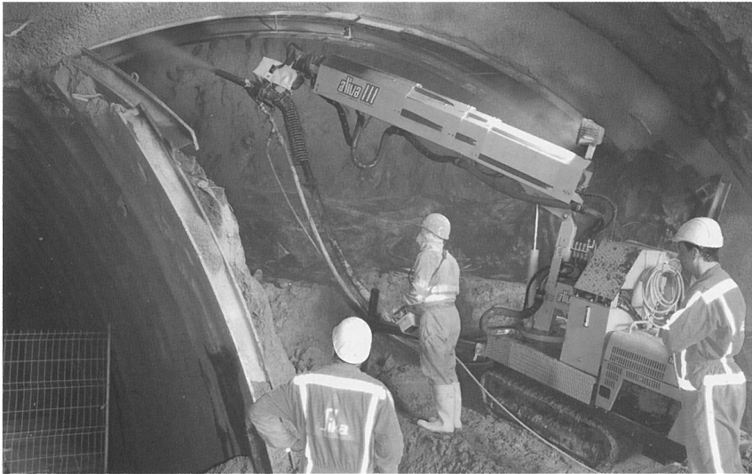
Fig. 38: sprayed concrete test for controlling rebound
