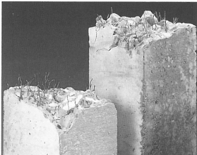
Fig. 18: failure surface of two prisms
