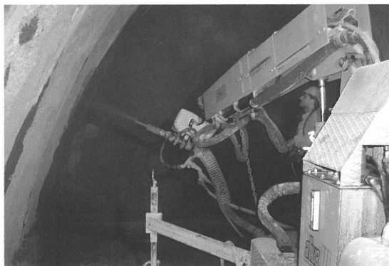
Fig. 3: wet spray application
