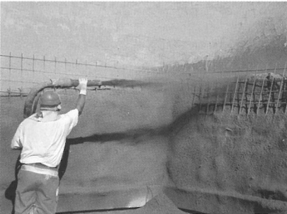
Fig. 26: nozzle man spraying manually
