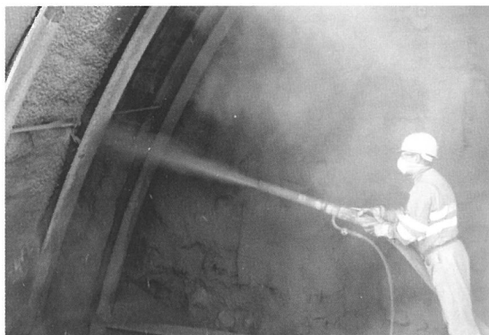
Fig. 2: dry spray application
